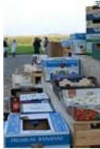
The new urban training area at Chièvres Air Base, Belgium, includes more than 30 buildings and an outdoor market. The area was built in less than three months to prepare soldiers, civilians and allied partners of the 650th Military Intelligence Group for their upcoming deployment. U.S. Army photo by Vanessa Thonnard, 7th U.S. Army Joint Multinational Training Command
